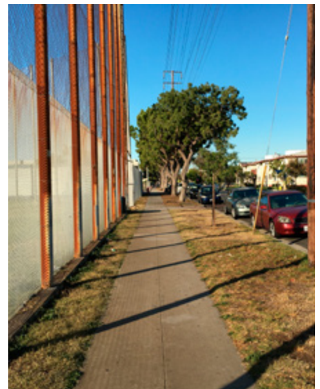
Parkway looking north on Inglewood Avenue
