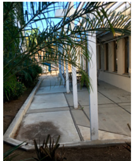
Imperial Library looking west towards back alley.
