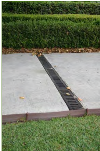
The driveway grate, an unobtrusive addition to the property, directs stormwater down into the underground drywell.
