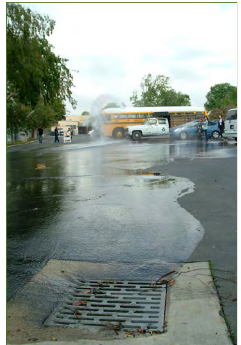
Water drains into a storm drain after a mock flash flood at Open Charter. Rather than running off the campus and eventually into Santa Monica Bay, stormwater is collected and detained onsite by a system of BMPs including trees, vegetation, swales and a cistern.
