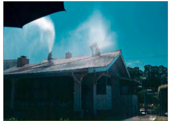
A mock storm “rained” 4,000 gallons onto the Hall House property during a demonstration following the project’s completion.
