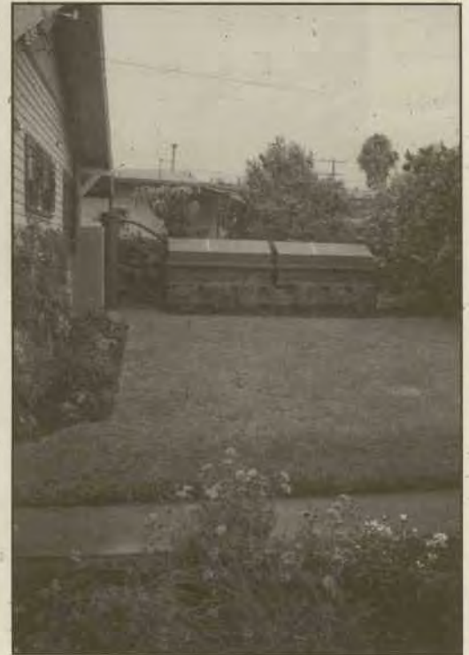
Rear yard of the demonstration site as it looks today. Grass panel holds, then absorbs, nearly 4,000 gallons of water. Two cistern units are visible at the far side of the yard. The cylindrical roof wash unit can be seen to the immediate left of the cistern. Roof water drains from the downspout into the roof wash unit, where impurities settle out. Clean water is decanted into cistern from the pipe connecting the top of roof wash unit to the top left corner of the cistern.
